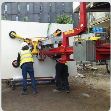
Libro 2500B fitted with a modified MRTA8 vacuum lifter on a manipulating head for installing GRC soffit panels
