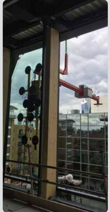
*Libro 2500B fitted with a modified MRTA8 vacuum lifter on a manipulating head for installing GRC soffit panels*
